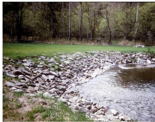
Butternut Creek After Stabilization
