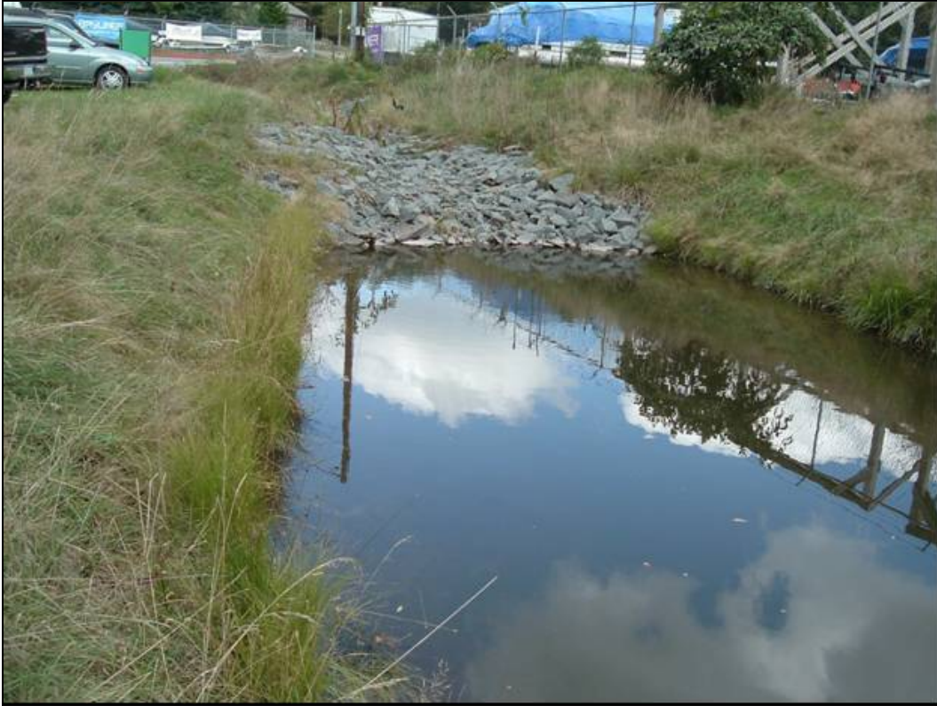
Sediment Forebay at Constructed Wetland Inlet – after BMP installation
