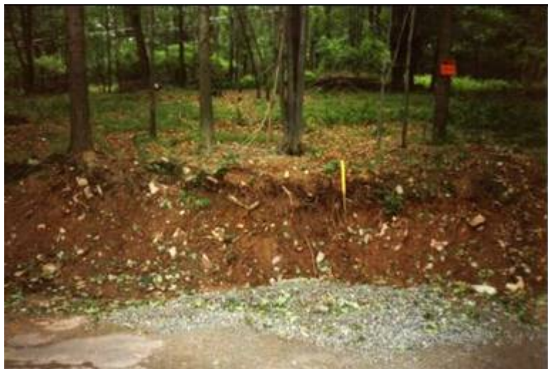
Roadside bank erosion problem area
