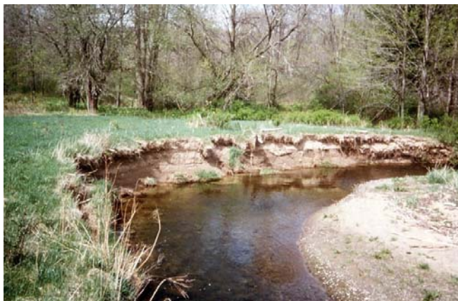
Butternut Creek Before Stabilization
