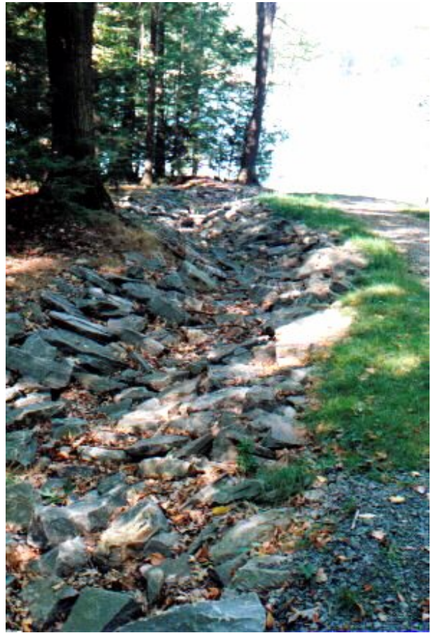
Rock-lined channel designed to reduce stormwater erosion along roadside in Paupack Township
