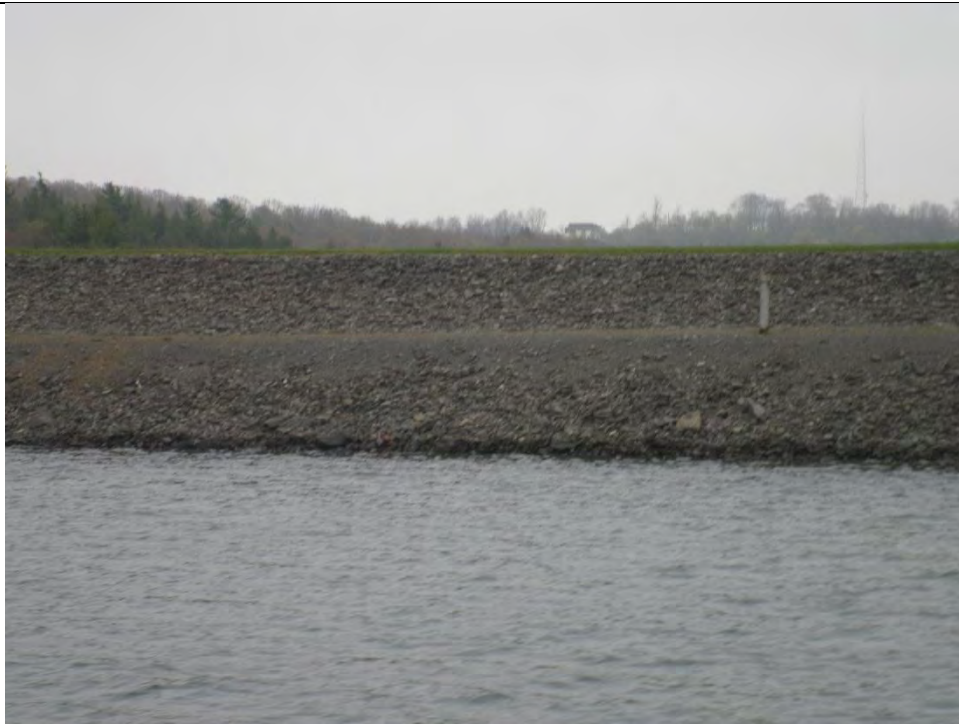
Photo #401 Close-up of Dam
