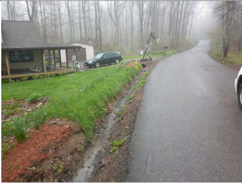
Photo #423 Roadside drainage ditch
