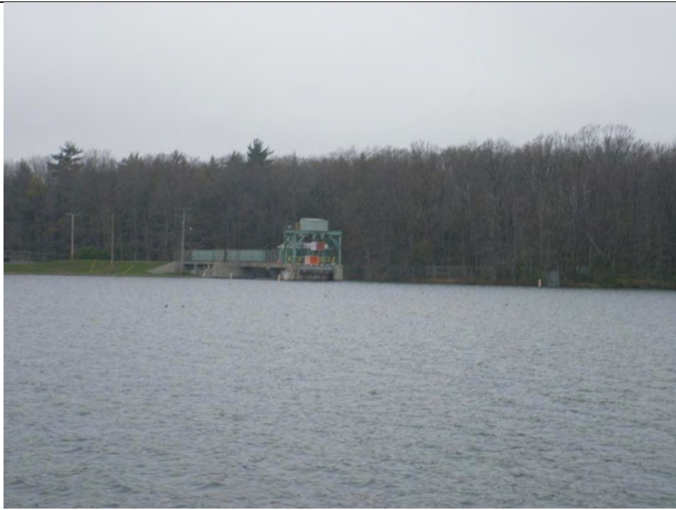
Photo #399 Hydroelectric Plant
