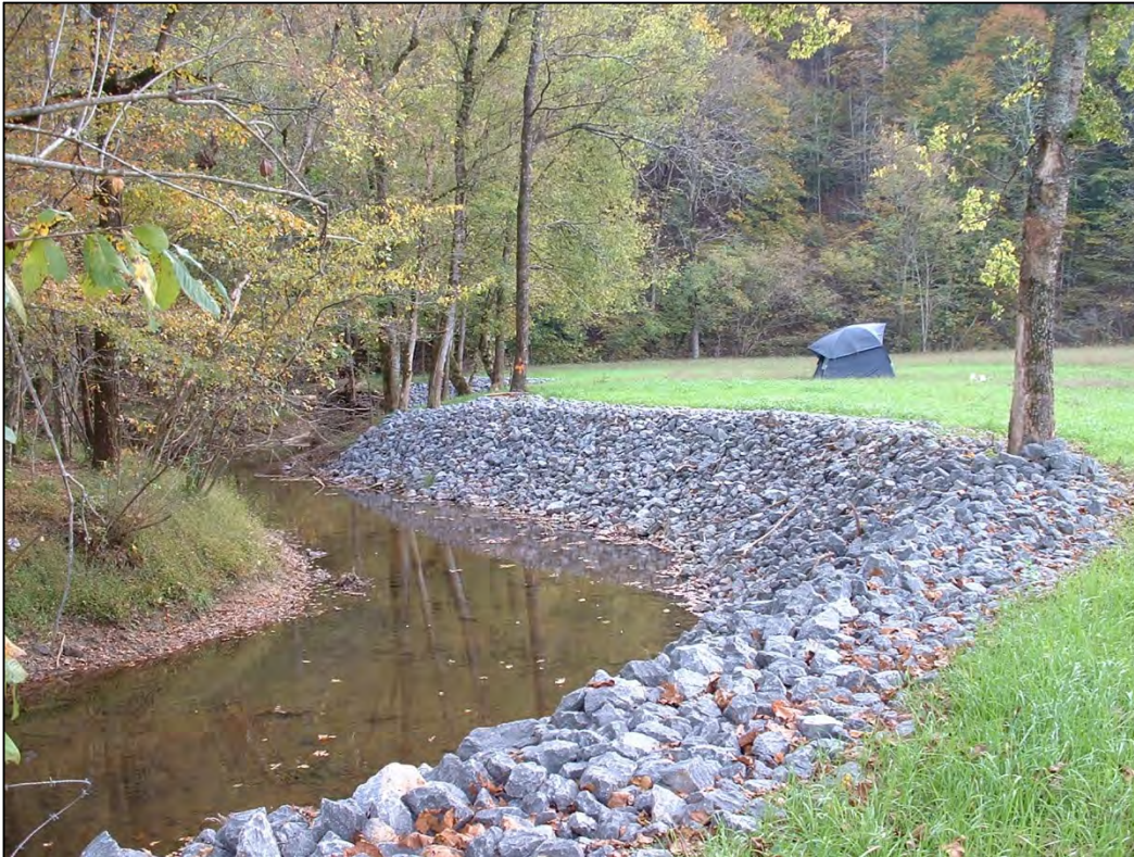
Figure 8: Riprap Used for Structural Stream Bank Stabilization
