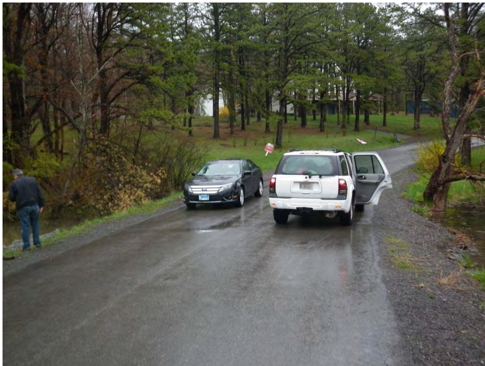
Photo #409 Typical public road – 2 lanes, no curb/gutter
