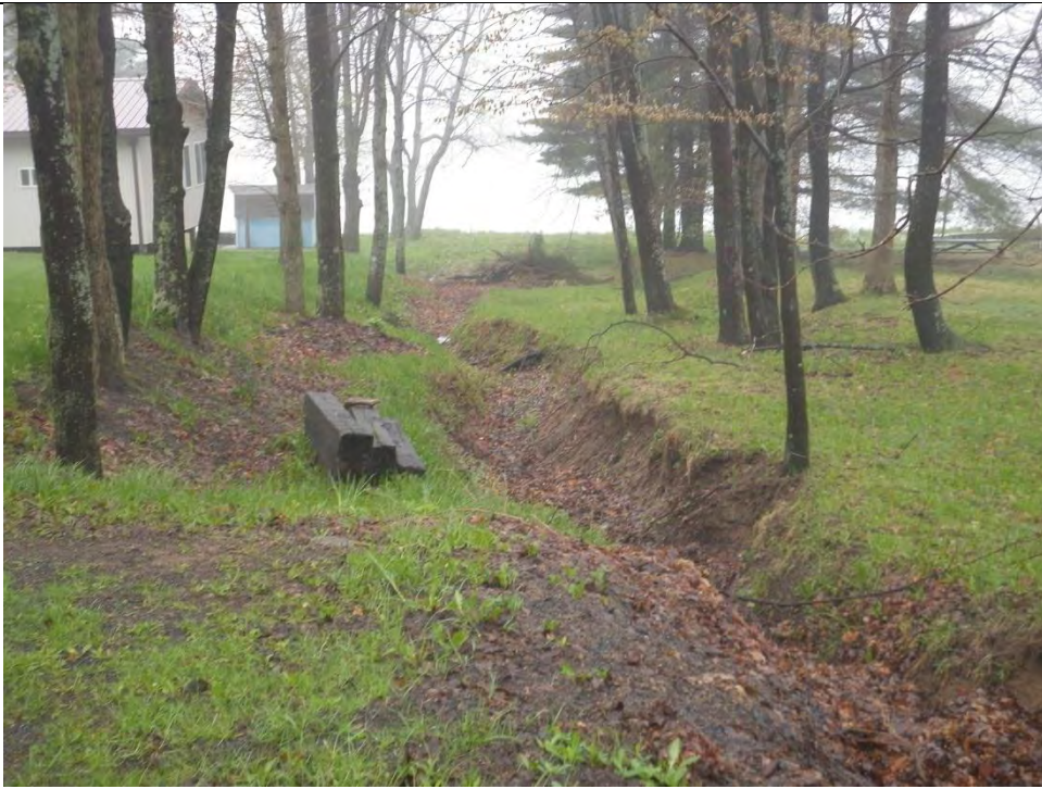
Photo #420 Roadside drainage ditch
