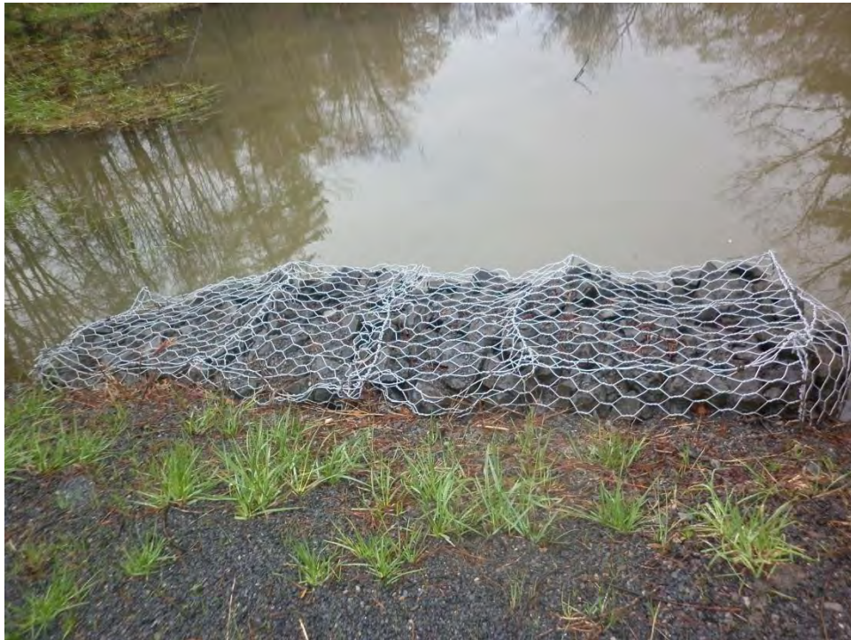
Photo #411 Gabion outlet protection
